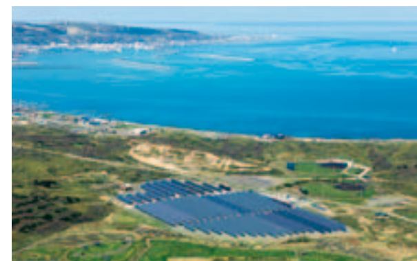
Experimental research facilities on a solar energy power plant in Wakkanai
